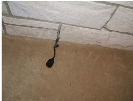
The wiring behind the fireplace needs to be removed and properly discontinued.
